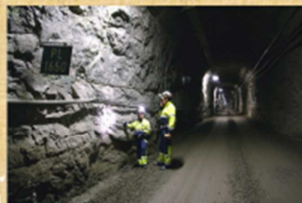
Access tunnel, 5 km
